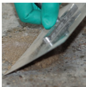
Filling cracks and crevices MC-DUR TopSpeed SC with sand filler
