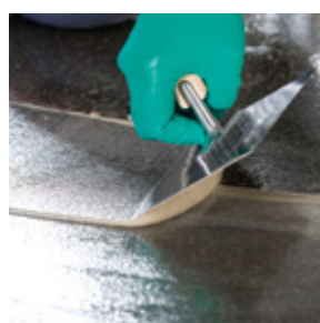
Scratch and levelling coat MC-DUR TopSpeed SC with sand filler
