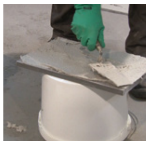
Adhesive coating over the full area
